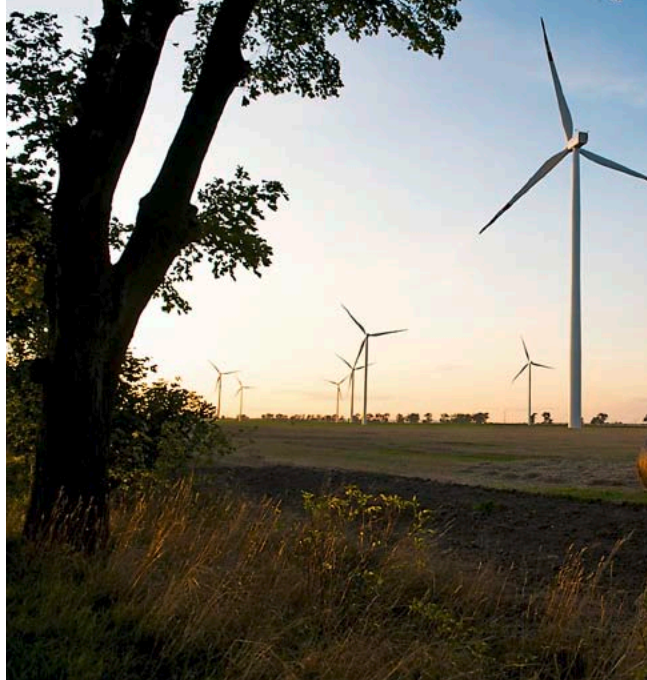
Lake Ostrowo wind farm, Wolin, Poland © Wind Power Works
