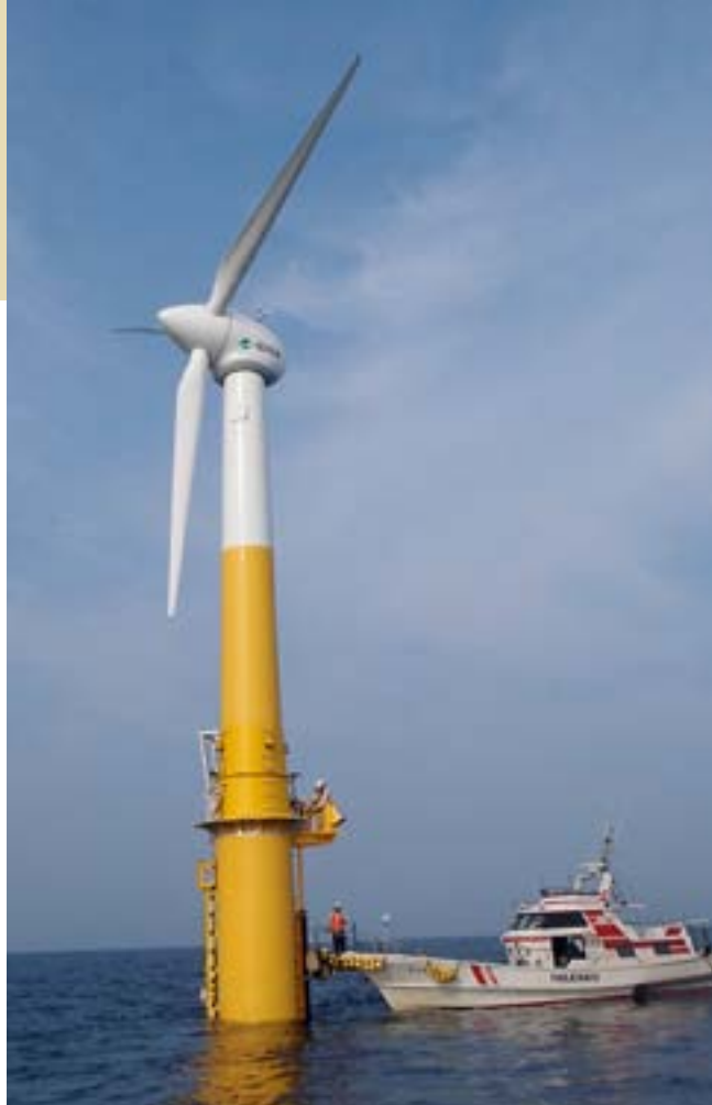
100 kW floating offshore wind turbine in Kabashima in Nagasaki Prefecture © MOE
