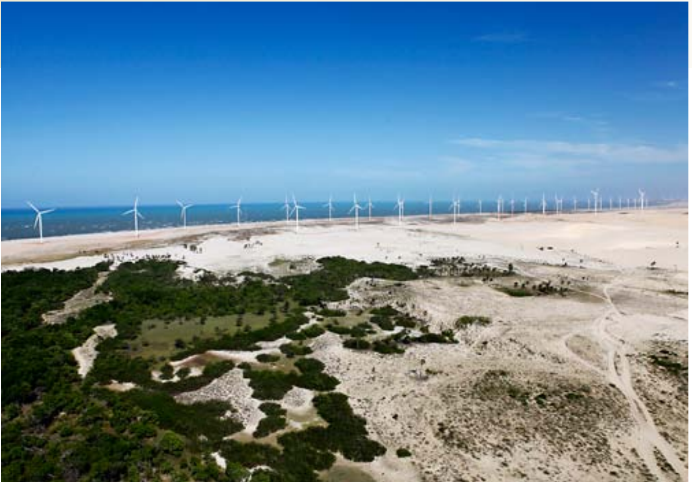
noa Quebrada Wind Farm, Ceará, Brazil © ABEEólica'
