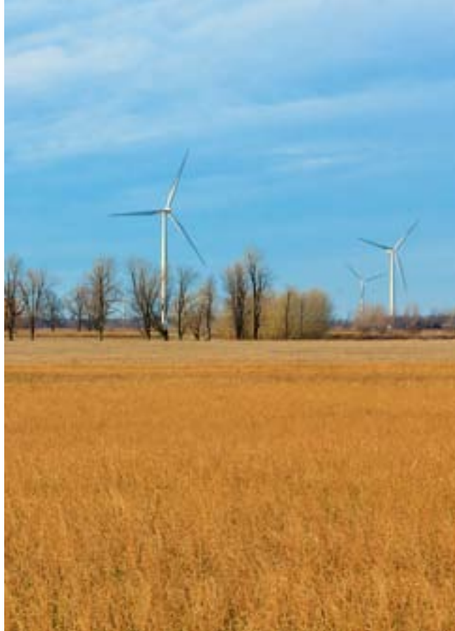
Wolfe Island wind farm, Kingston, Ontario © Canadian Wind Energy Association
