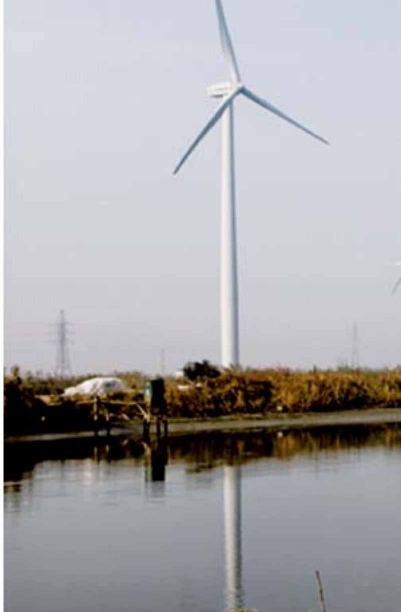
Xiao Yan Kau wind farm, Rudong © Wind Power Works
