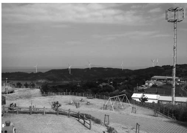
Azuchi Oshima wind farm, Nagasaki Prefecture © M&D Greenenergy Co. Ltd
