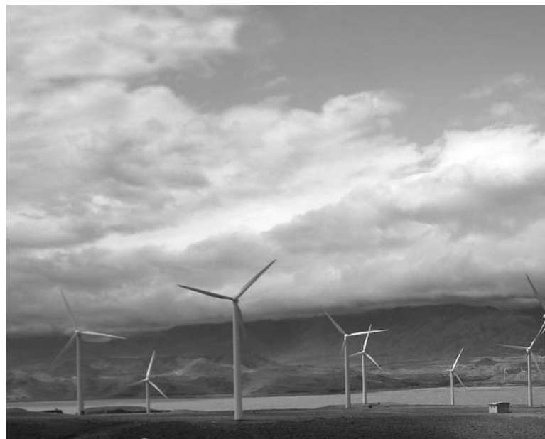
Manjil wind farm, Guilan © Saba Niroo Co. Wind Turbines & Power Plants
