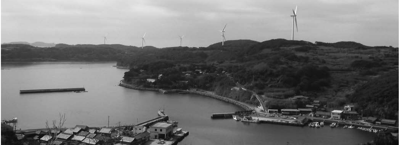
Azuchi Oshima wind farm, Nagasaki Prefecture © M&D Greenenergy Co. Ltd
