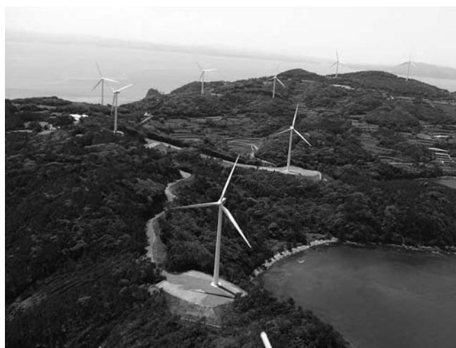
Azuchi Oshima wind farm, Nagasaki Prefecture © M&D Greenenergy Co. Ltd
