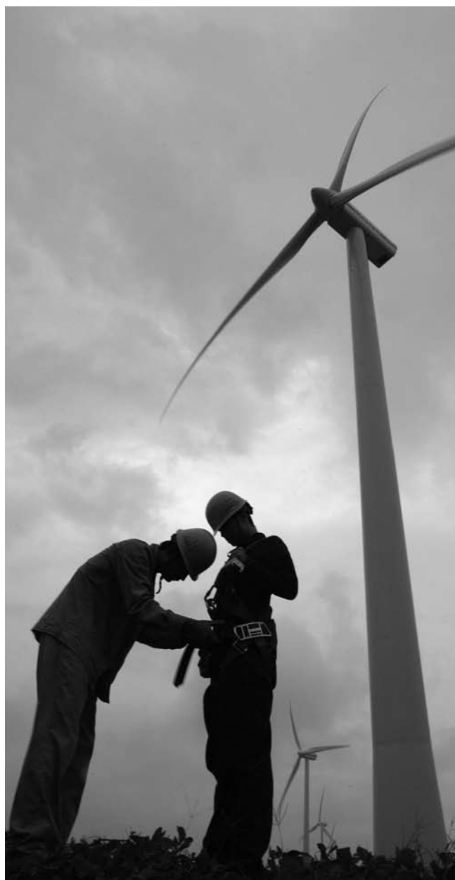
Fujian Dongshan Wujiao Wan wind farm, Dongshan, Fujian
