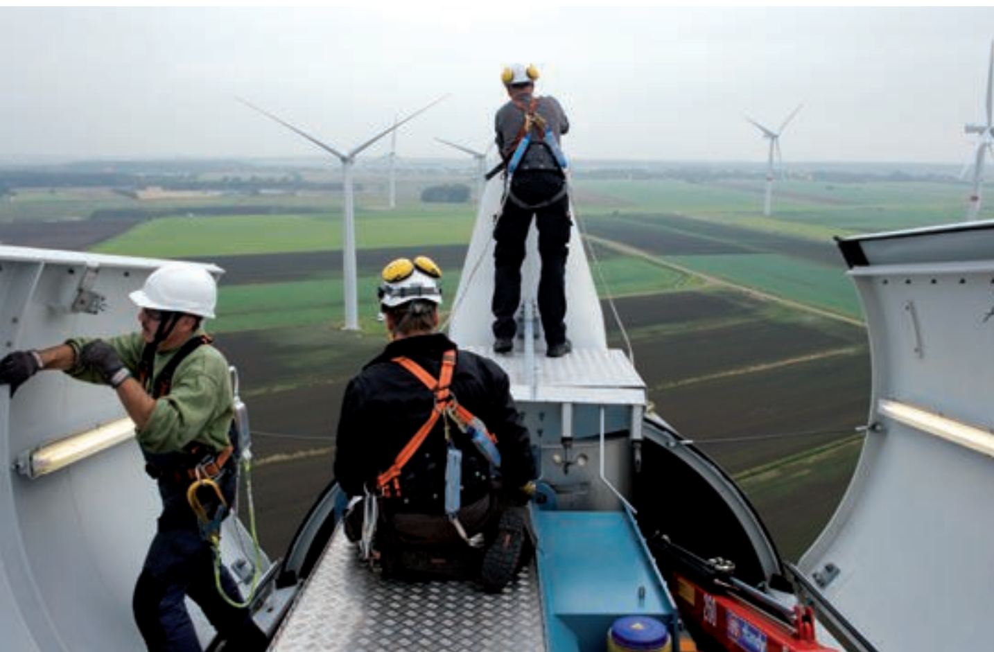
Germany, Marienkoog wind farm (Photo: Wind Power Works)
