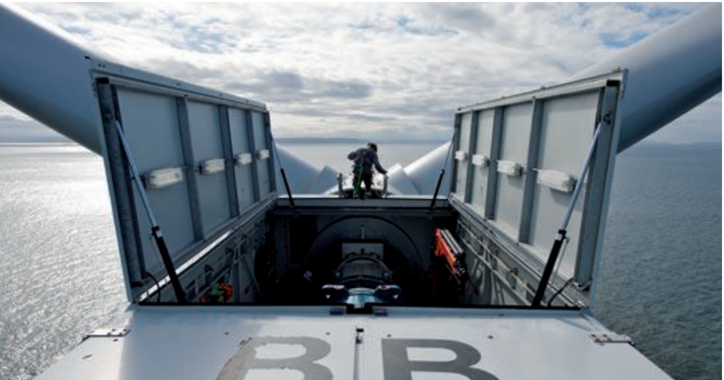
Burbo Bank wind farm (Photo: Wind Power Works)
