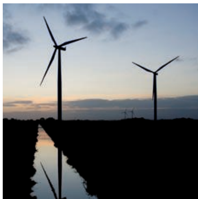
Germany, Marienkoog wind farm (Photo: Wind Power Works)
